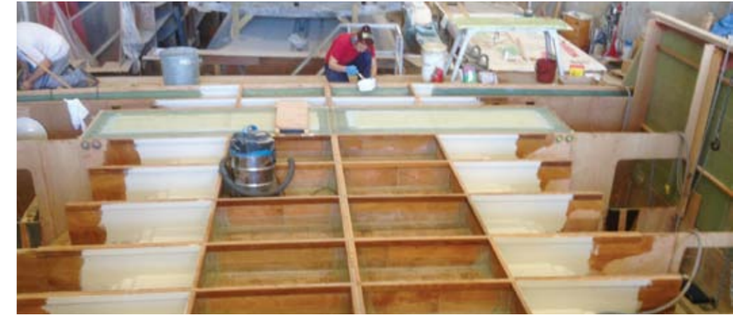
Wingdeck structural grid under aft deck.
