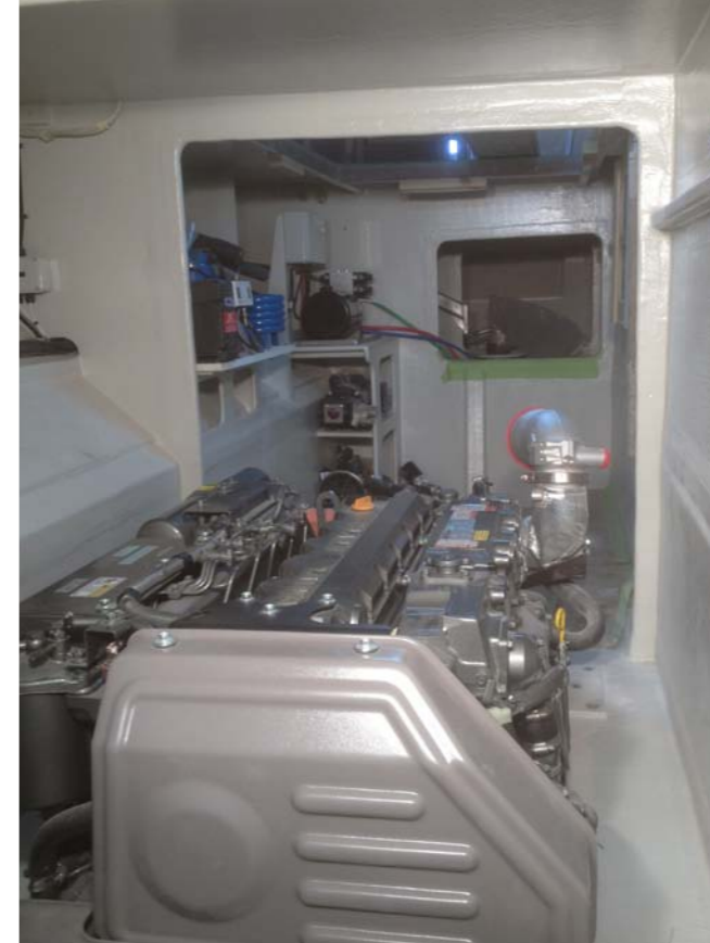
The engineroom is laid out in such a way as to be easily accessible for both operation and maintenance.
